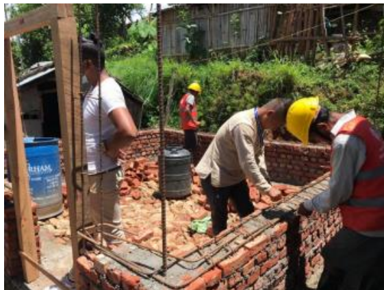
ANS handholding onsite mason training at Gorkha NP
