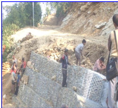
Gabion wall works at Tandarnj VDC, Gorkha
