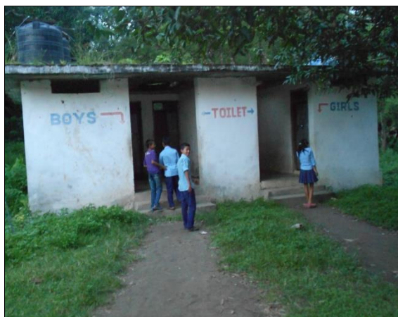
School Toilet in Aarughat water supply & sanitation Scheme at Aaruchanaute VDC, Gorkha
